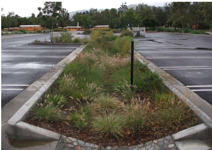
Figure 19: Bioswale Source: http://bit.ly/silverfigD3
