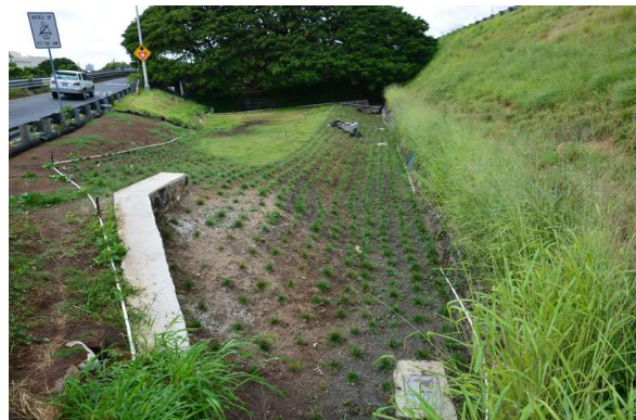
Figure 11: For the Ala Wai Watershed Storm water BMPs on Oahu Project, median areas between the freeway off ramps, were converted into bioswales. The bioswales consist of an under drain system, which includes a perforated drain pipe and engineered soils that provide filtering. Above this, native vegetation was planted to slow and filter storm water as it first enters the bioswales. Additionally, the design includes an outfall structure that forces storm water to pond in the median allowing more time for infiltration into the under drain or evaporation.
