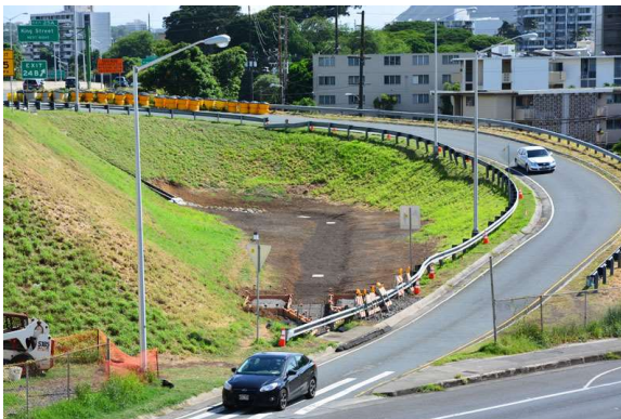
Figure 11: For the Ala Wai Watershed Storm water BMPs on Oahu Project, median areas between the freeway off ramps, were converted into bioswales. The bioswales consist of an under drain system, which includes a perforated drain pipe and engineered soils that provide filtering. Above this, native vegetation was planted to slow and filter storm water as it first enters the bioswales. Additionally, the design includes an outfall structure that forces storm water to pond in the median allowing more time for infiltration into the under drain or evaporation.
