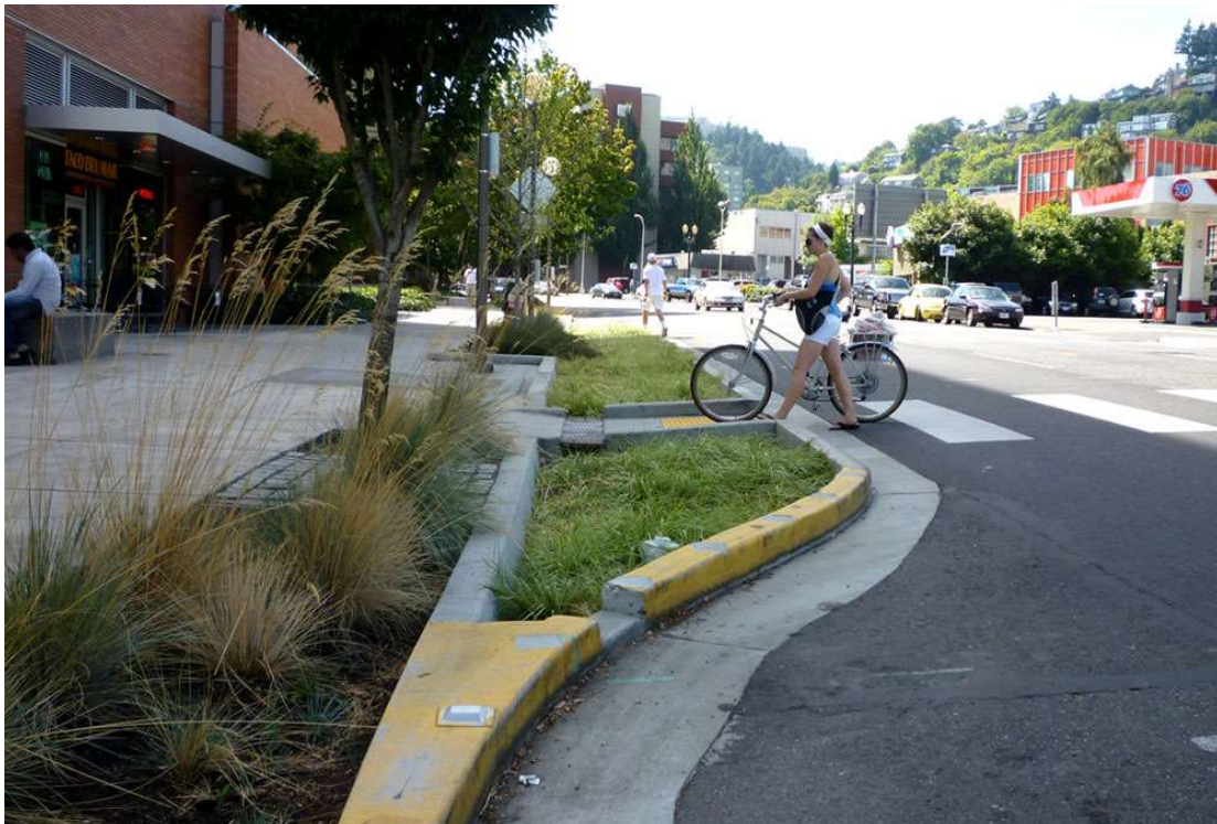
Figure 15: Sustainable Jersey awarded the City of Hoboken a Sustainable Jersey Small Grant for rain garden curb extensions. Rain garden curb extensions will help New Jersey reach set sustainability goals of alleviating flooding by capturing stormwater runoff and further promoting walking through safer pedestrian crossings
