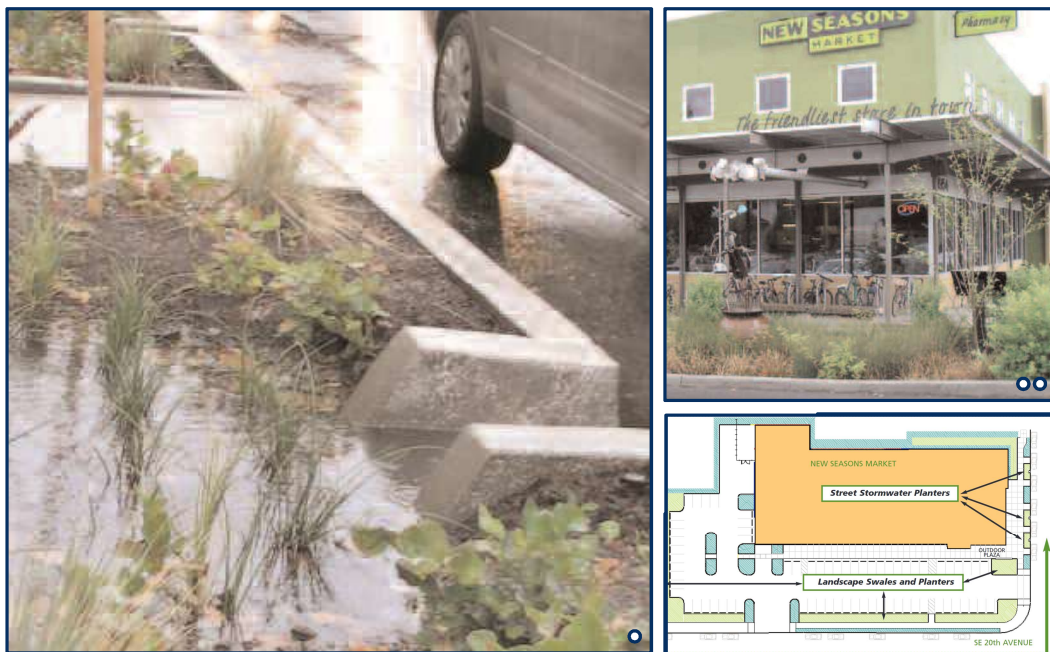
Figure 13: New Seasons Market in Portland, Oregon, installed a ring of interconnected storm water swales. Three storm water planters within a 6-foot planting strip between the sidewalk and street curb slows and filters runoff from Division Street.
